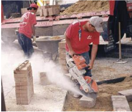
Dry sawing concrete
