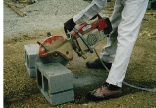
Wet sawing concrete water is added at saw blade
